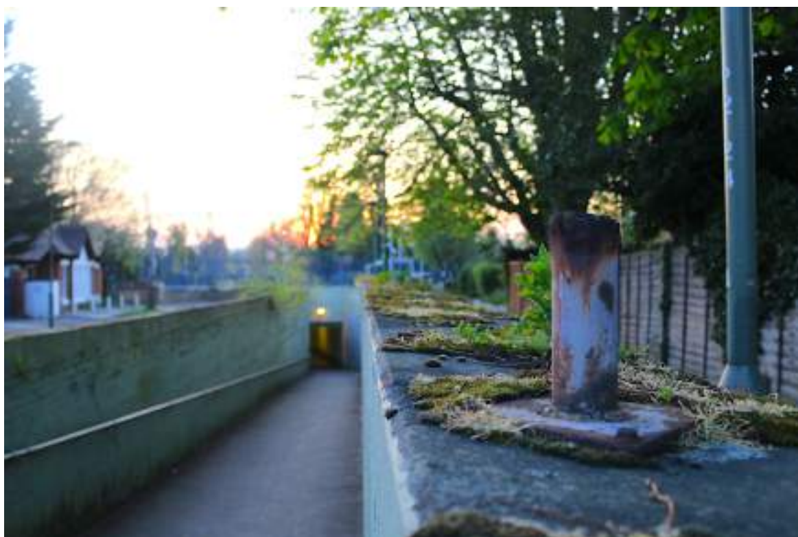
Miniature gardens on the passageway, growing from the concrete.
